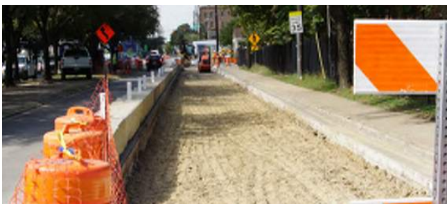
Construction on Navigation Boulevard Roundabout - East End District
