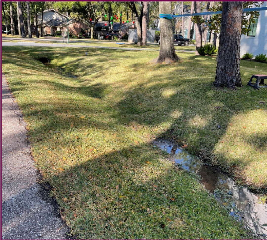
Figure 3. High point in ditch.
