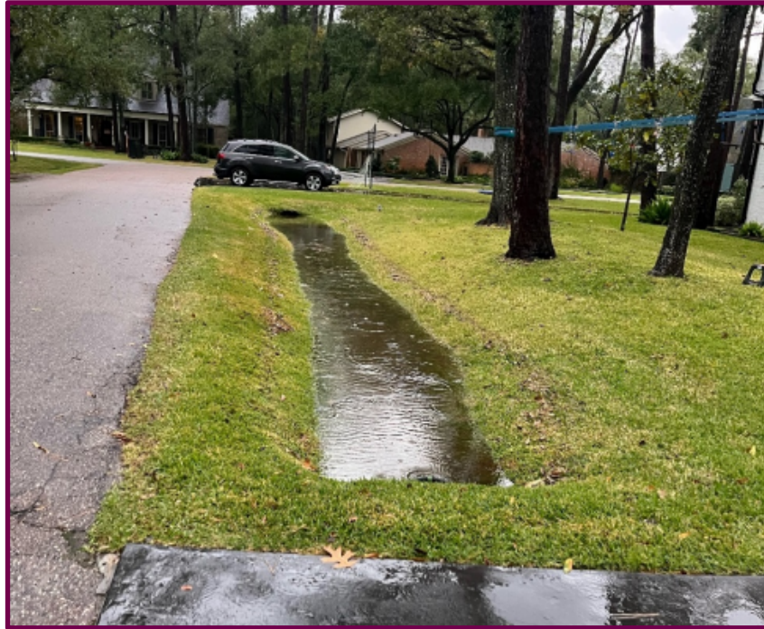
Figure A.1. Resident Picture of Williamsburg Ditch during a storm.
