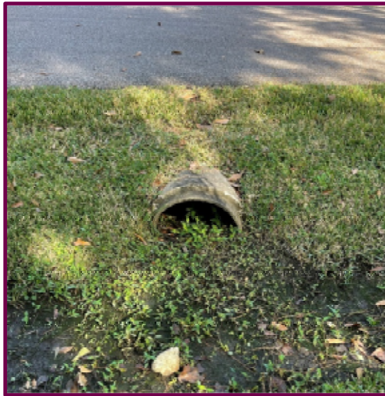
Figure 4. Silted in culvert across Williamsburg Lane
