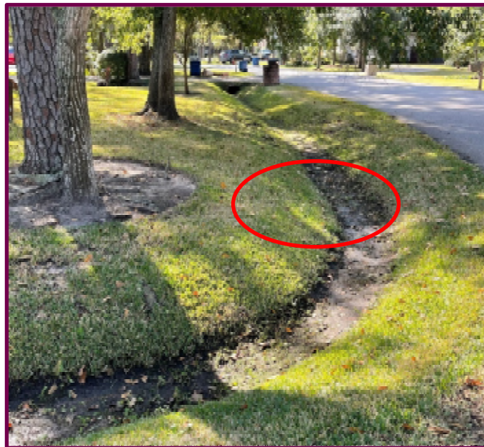
Figure 4. Silted in culvert across Williamsburg Lane
